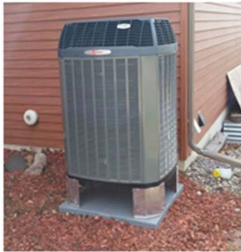
Whole home ducted cold-climate air source heat pump
