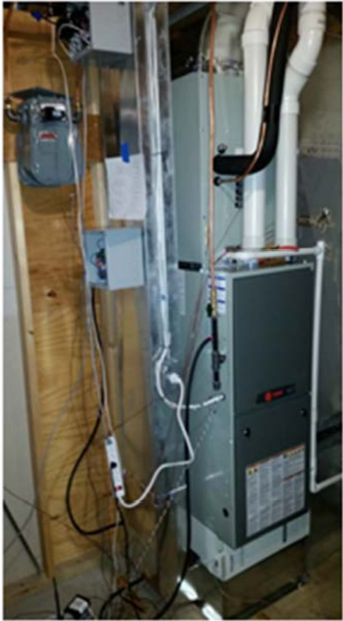
Whole home ducted cold-climate air source heat pump
